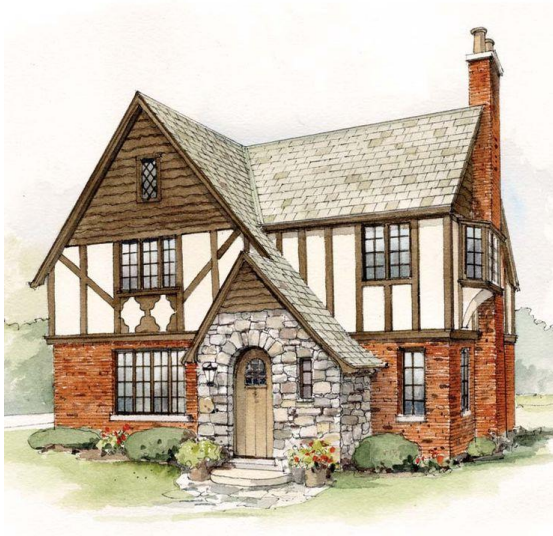
Exposed Timbering Filled with Plaster
